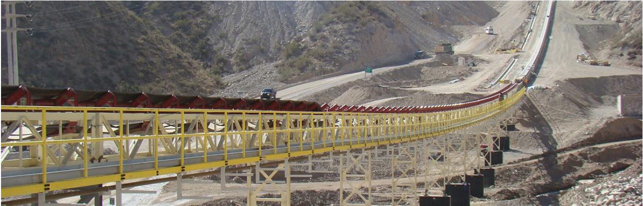
Conveyors will greatly reduce dust from the mine by cutting the number of trucks required
