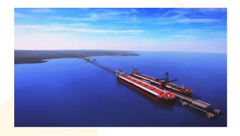
Capesize and Panamax capable, with additional module offloading facility (MOF).
