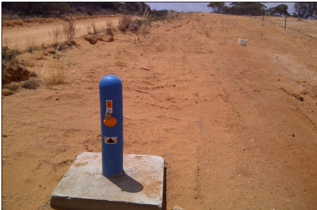
Figure 3 Capped groundwater monitoring hole east of Murphy Road.
